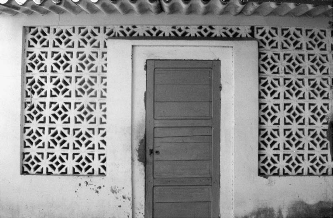
Figure 7. Women's prayer building screened by claustra work. Thies, Senegal. Photo Credit: Cleo Cantone.
